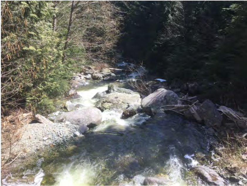
Looking downstream from deck
