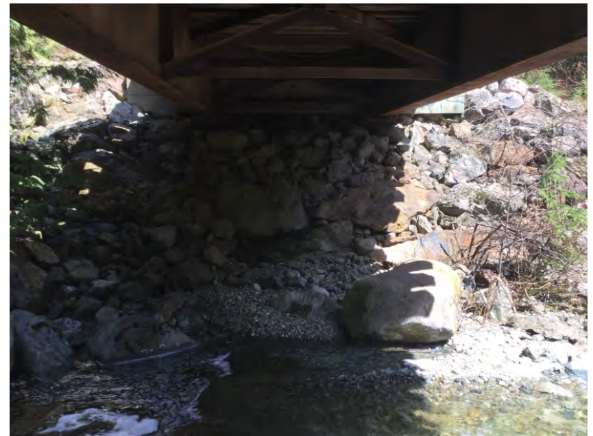
Left Bank Abutment when facing downstream
