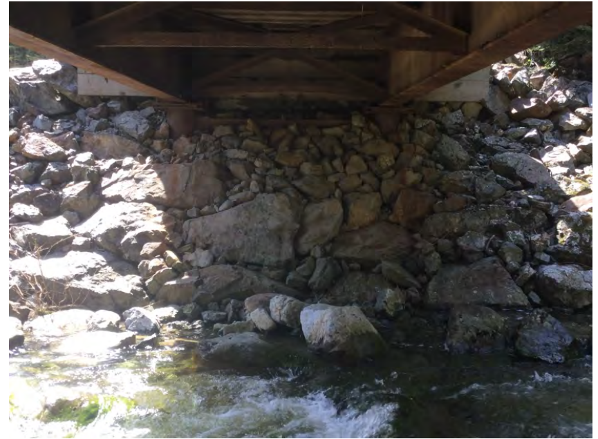
Right Bank Abutment when facing downstream
